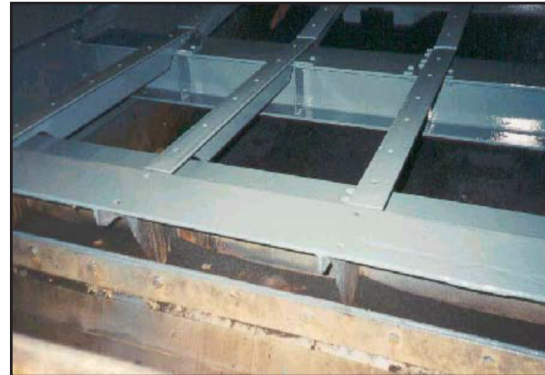
ARC S2 grey applied to coal screen
