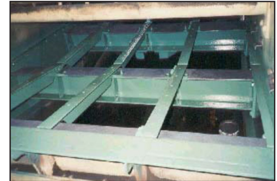
ARC BX2* applied to top rails
